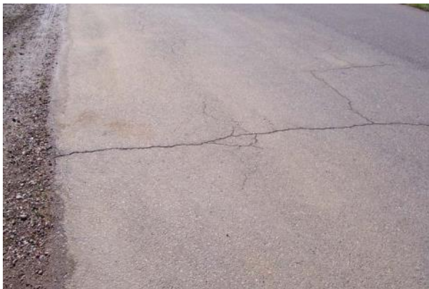
Transverse Crack
