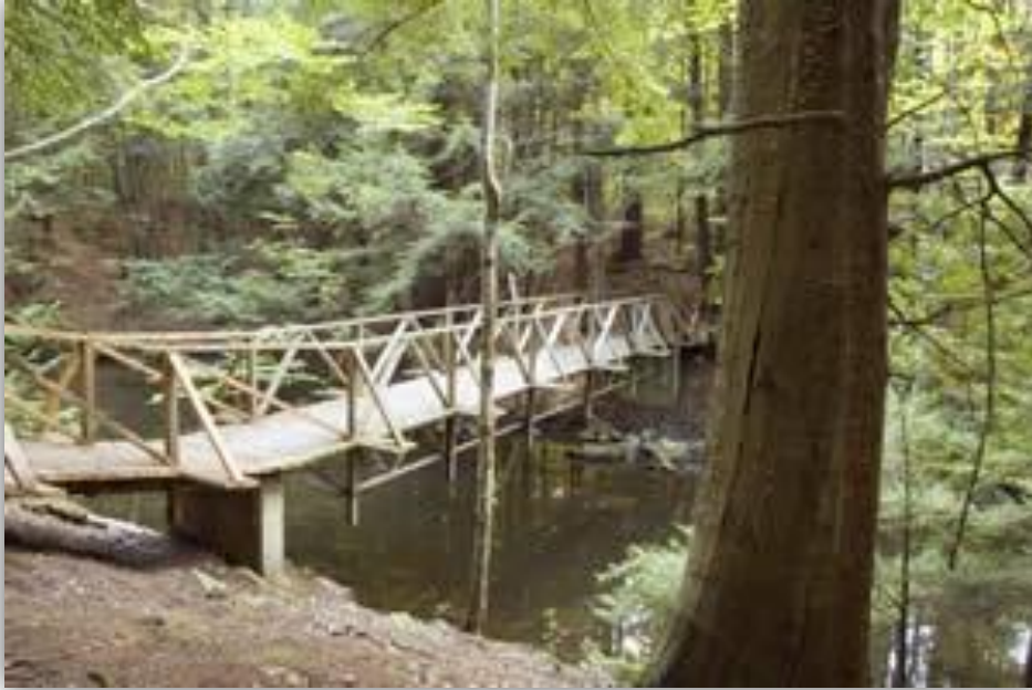
Footbridge in College Woods
