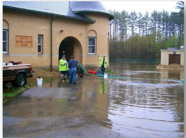
Wastewater Treatment Facility – 2006 Flooding Event
