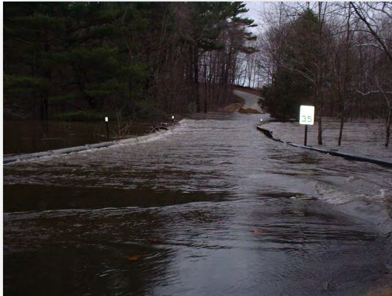
High Road Bridge, May 2006 Flooding Event
