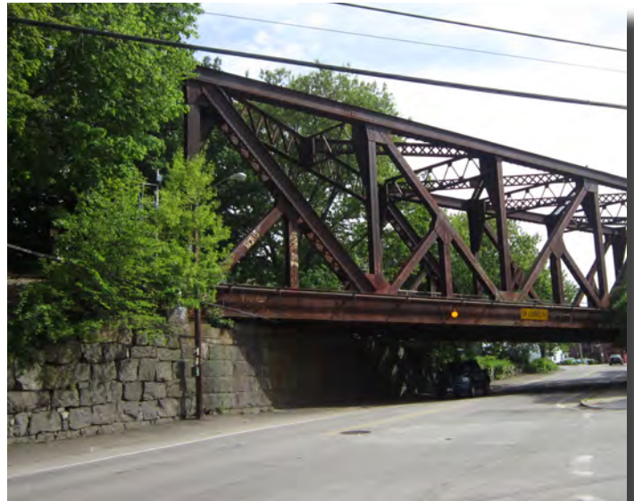
Bridge over Broadway St. in Dover Source: SRPC
