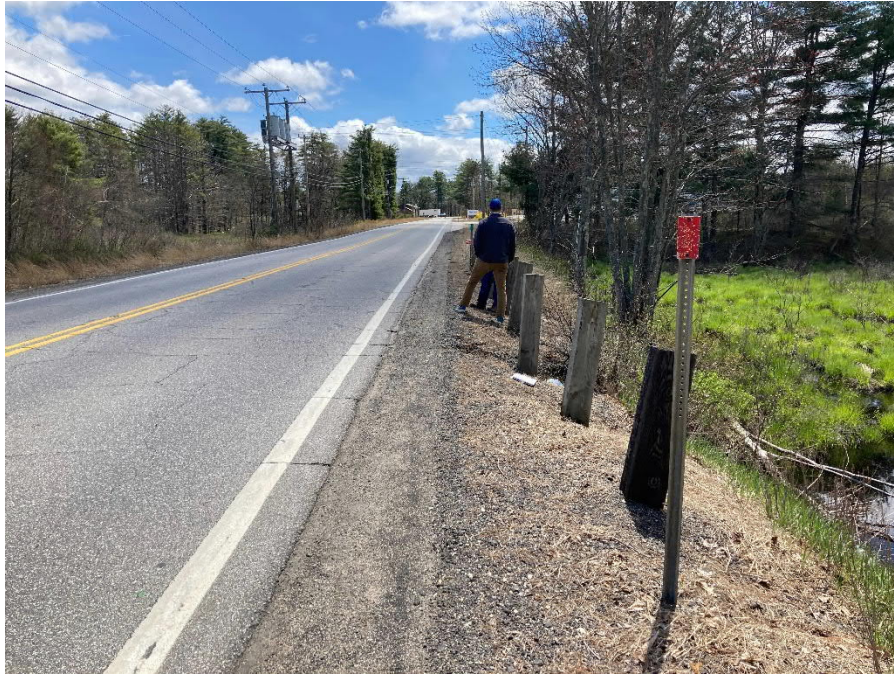
Main Street (Canal to Rec. Trail) – Crossing at Pokamoonshine Brook
