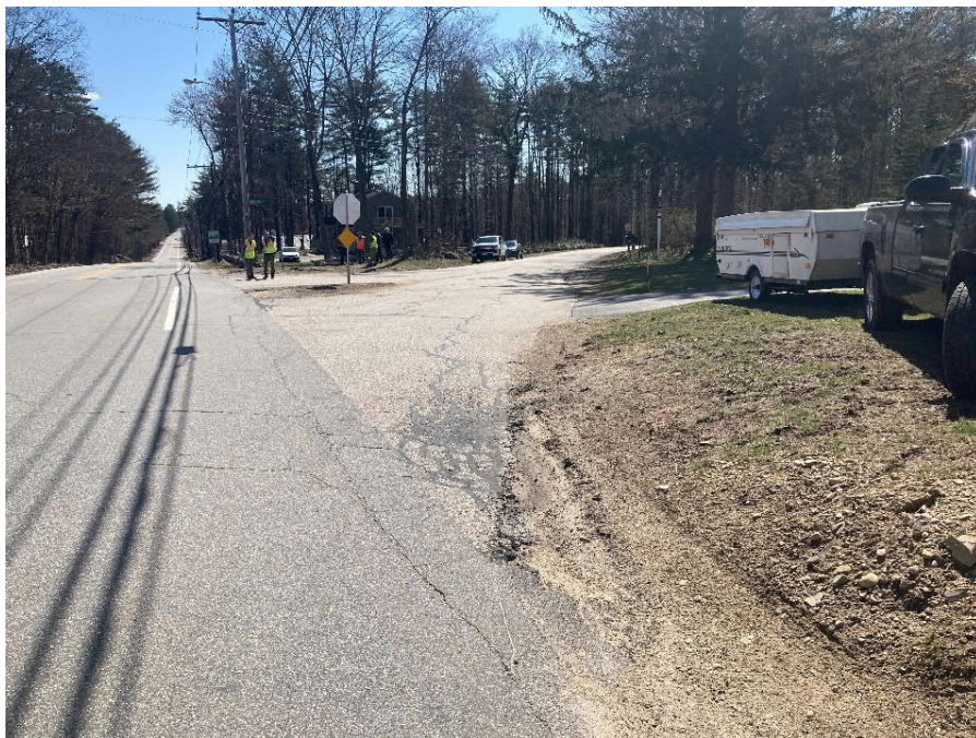
Departure lane from Route 9 to Old Stage Road
