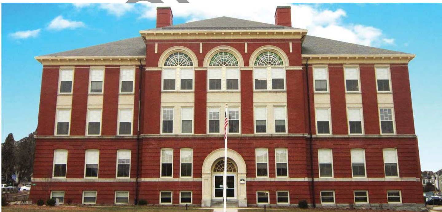
Location of the Dover Adult Learning Center at the McConnell Center, Dover Source: SRPC
