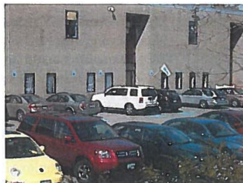
Main Office Entrance
