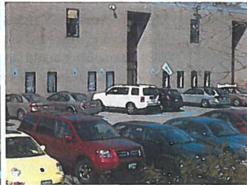
Main Office Entrance
