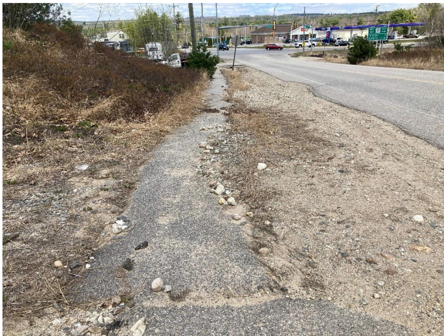
Main Street (Canal to Rec. Trail) – Existing sidewalk from Rte. 11 to Rec. Trail
