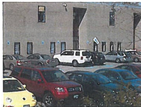
Main Office Entrance
