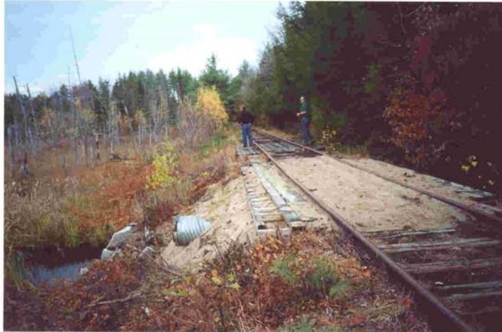
Fig. 2: Temporary culvert replacement
